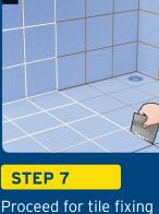
Proceed for tile fixing with Dr. Fixit/Roff tile adhesive and tile grouts to fill the tile gaps.
