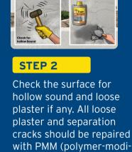
fied mortar) at the cement: sand ratio of 1:3 using Dr. Fixit Pidicrete URP 10% by weight of cement.
