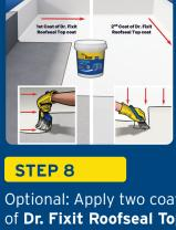
Optional: Apply two coats of Dr. Fixit Roofseal Top Coat, without water dilution, that has Solar Reflectance Index (SRI) value 106 and reduces surface temperature up to 10°C\*\* in the peak summer.
