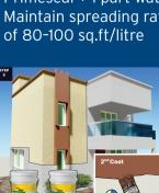
STEP 5 Apply second coat of Dr. Fixit Raincoat Classic Topcoat/Raincoat Select Top Coat in interval of 6-8 hrs without any dilution. Maintain spreading rate of
