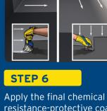
resistance-protective coating of Dr. Fixit Coal Tar Epoxy @ 26 sq.ft/Kg for 2 coats. It has excellent resistance to abrasion and a wide range of acids, alkali and salt solutions, effluents and sewage.
