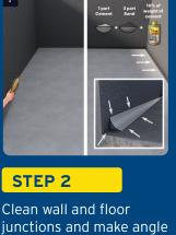
fillet/watta with cement: sand mortar (1:3) admixed
